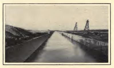
The Drainage Canal—Seventeen Miles of the Canal are Sawed Out of the Solid Rock
