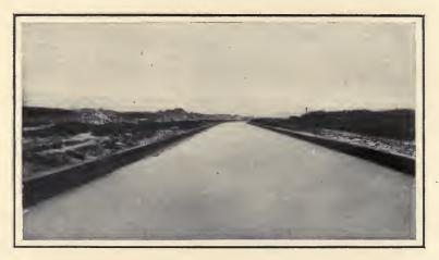
The Drainage Canal-Walls of Solid Stone Artificially Laid
